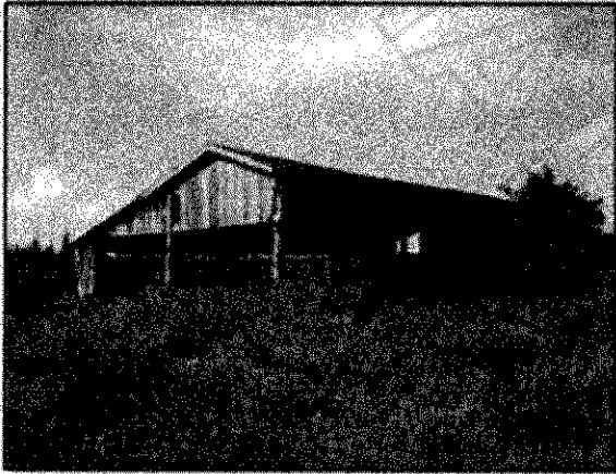
#3- Obsolete barn situated near the NE corner of P28865.
