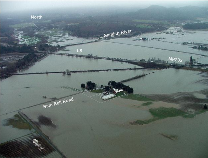
Figure 8.10 I-5 Flooding in Samish River north of Burlington during the flood of Jan 2009 (Source: URL 12).
