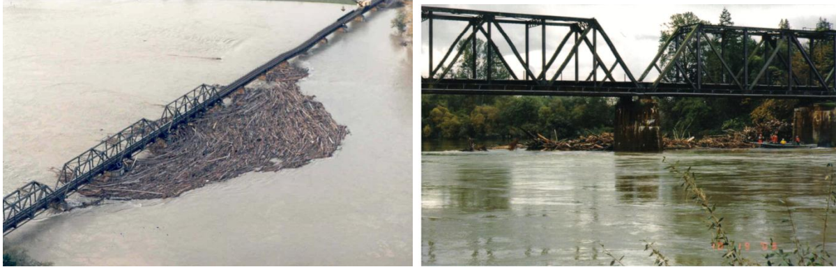
Figure 8.11 Log jams behind the Burlington Northern Railroad Bridge in November 1995 flood (left panel) and in October 2003 flood (right panel) (Source: URL 10).
