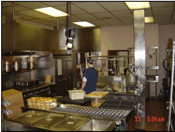
Figure 9.24 Kitchen Prep Area
