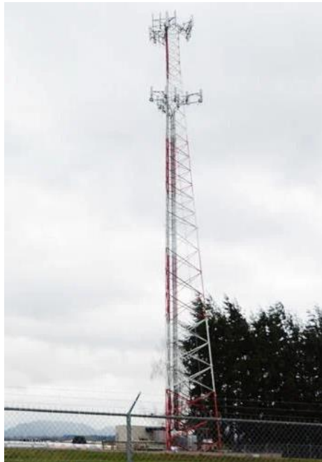
Figure 1 Macro Cell Tower
