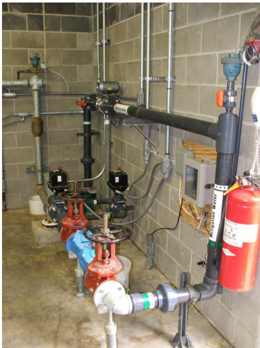
Picture 1- Well S02 in treatment house
