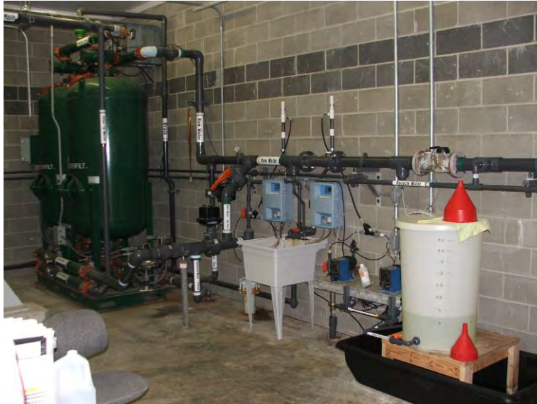
Picture 2 - Treatment house
