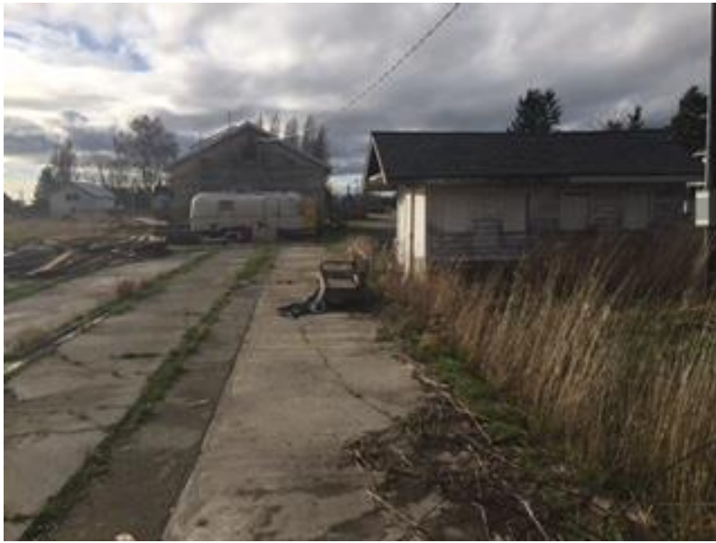
Looking westerly, with granary building in the back
