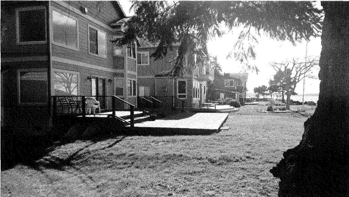
Current building codes require the main floor at a higher elevation than the ground line. This home shows the typical stairs required to get to the main floor elevation with currently building codes.
