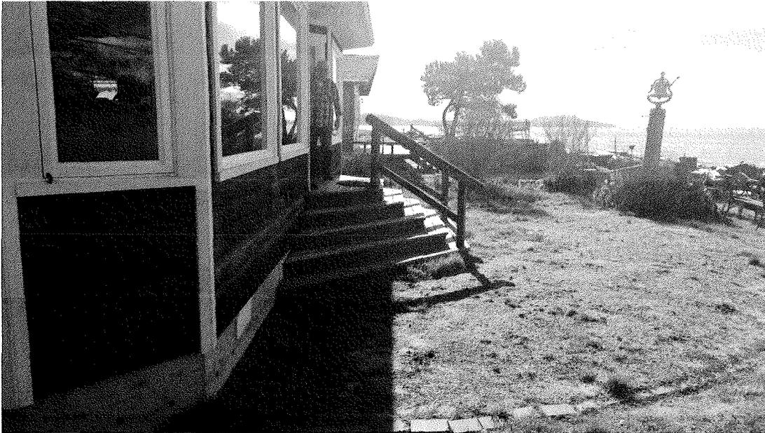
The existing Madden Home. Building codes require a new floor height about a foot higher than the bottom of the windows. The building envelope requires the home to be more narrow, no second story master bedroom, no side gable providing front roof overhang, and more out of scale to the neighboring homes.
