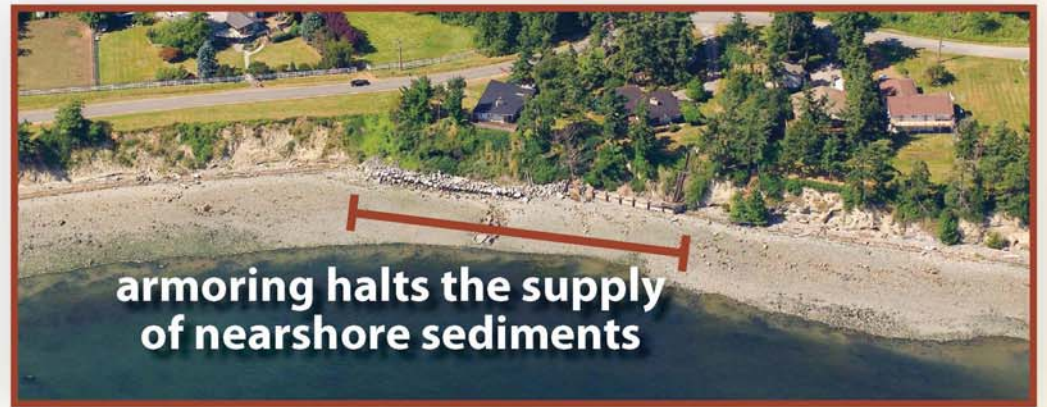
Upland development, including need to protect existing structures, can lead to unintended impacts.
