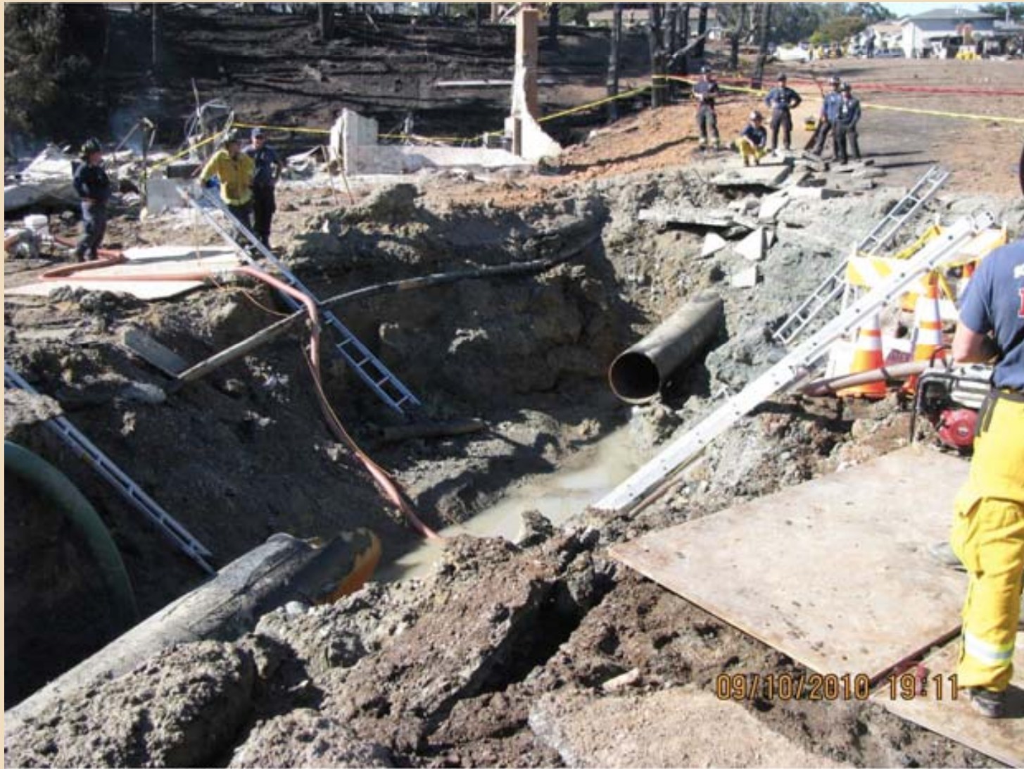
Exhibit 2CV: Pipeline Rupture Site Looking North, 10 Sept 2010 IMG_0097 NTBB Downs
