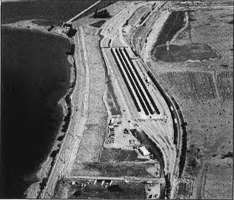
Figure 5. Aerial Photo Showing Tesoro's Newly Completed Rail Yard.
