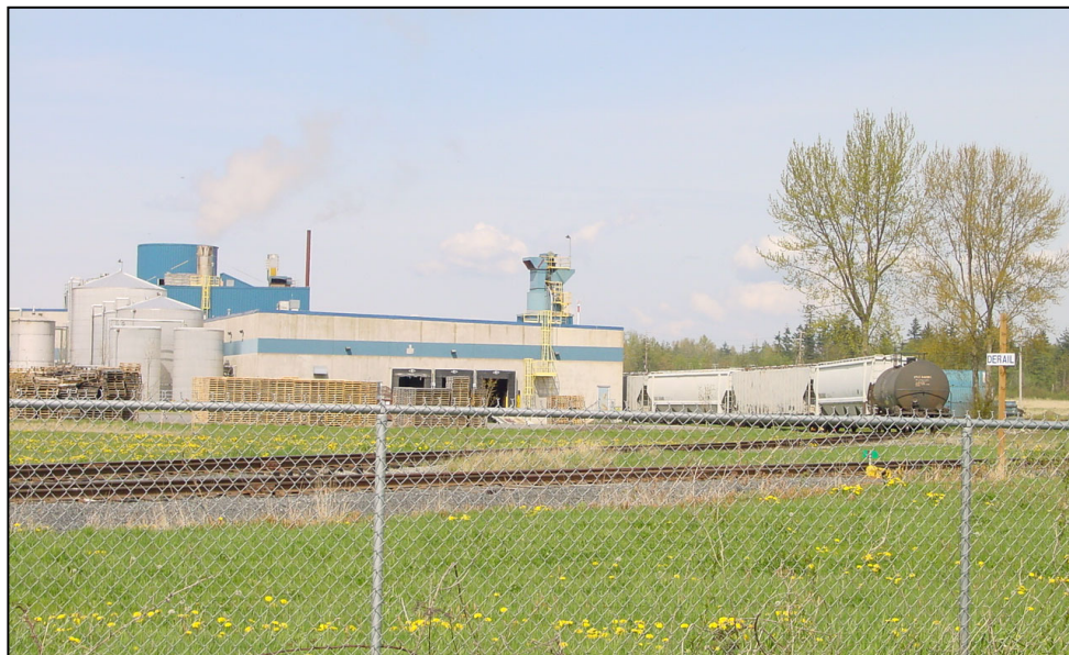
Bayview UGA Industrial Park
