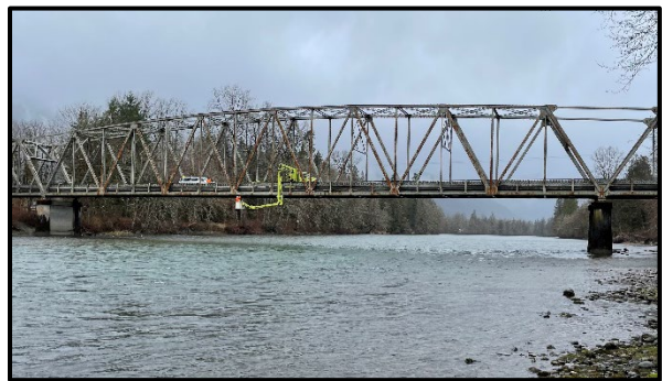
Skagit River Marblemount Bridge, UBIT inspection
