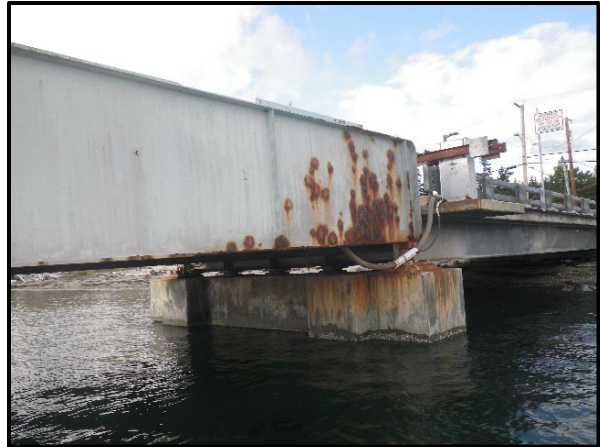
M/V Guemes Ferry Anacortes Terminal – Transfer Span
