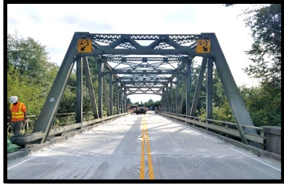
Samish River Bridge - Vertical Clearance Signage
