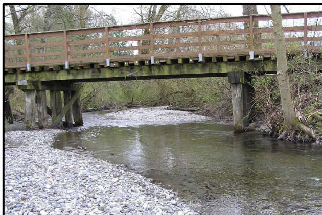
Cascade Trail Bridge at Jones Creek
