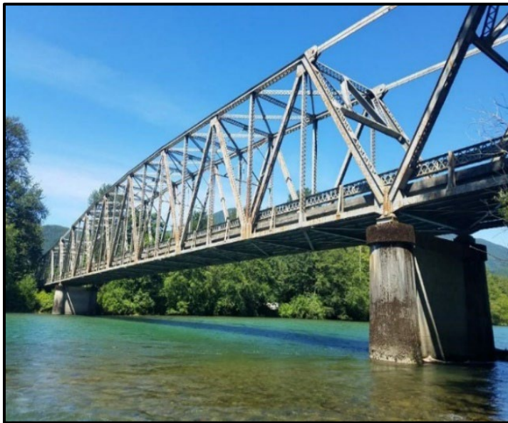
Marblemount Bridge – Skagit River
