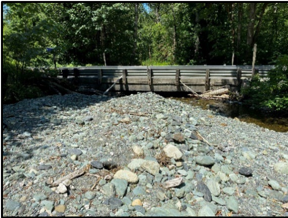
Mill Creek channel upstream of bridge.
