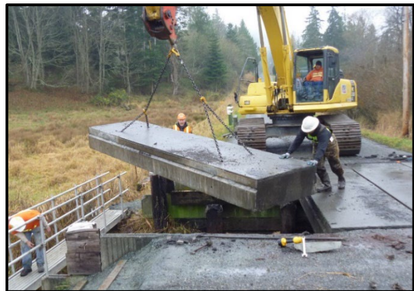
Campbell Lake Outlet receiving new timber cap in 2013
