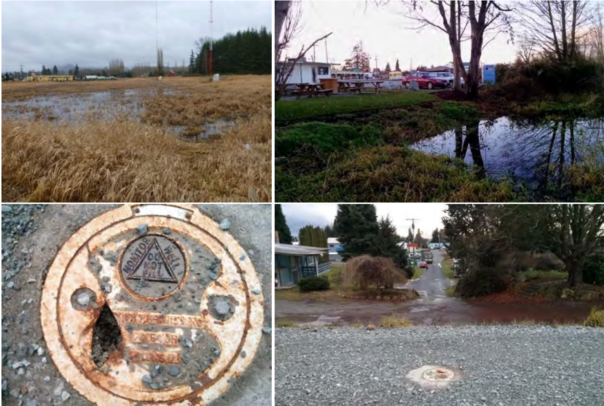
Figure 10: Photos of Monitoring Locations; (upper left, radio tower depression on south side of Highway 536; upper right, depression on north side of Highway 536; bottom left and bottom right, monitoring well on top of levee)
