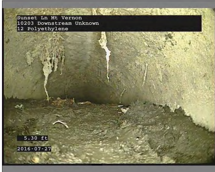
Photo: 10203Unknown27072016_120247.JPG 5.31FT, Deposits Settled Fine, 60 %of cross sectional area, from 03 to 09 o'clock, , within 8 inches of joint: NO
