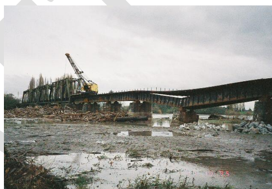
Figure 4a and 4b: Debris accumulation on the BNSF Bridge during 1995 flood event looking upstream.
