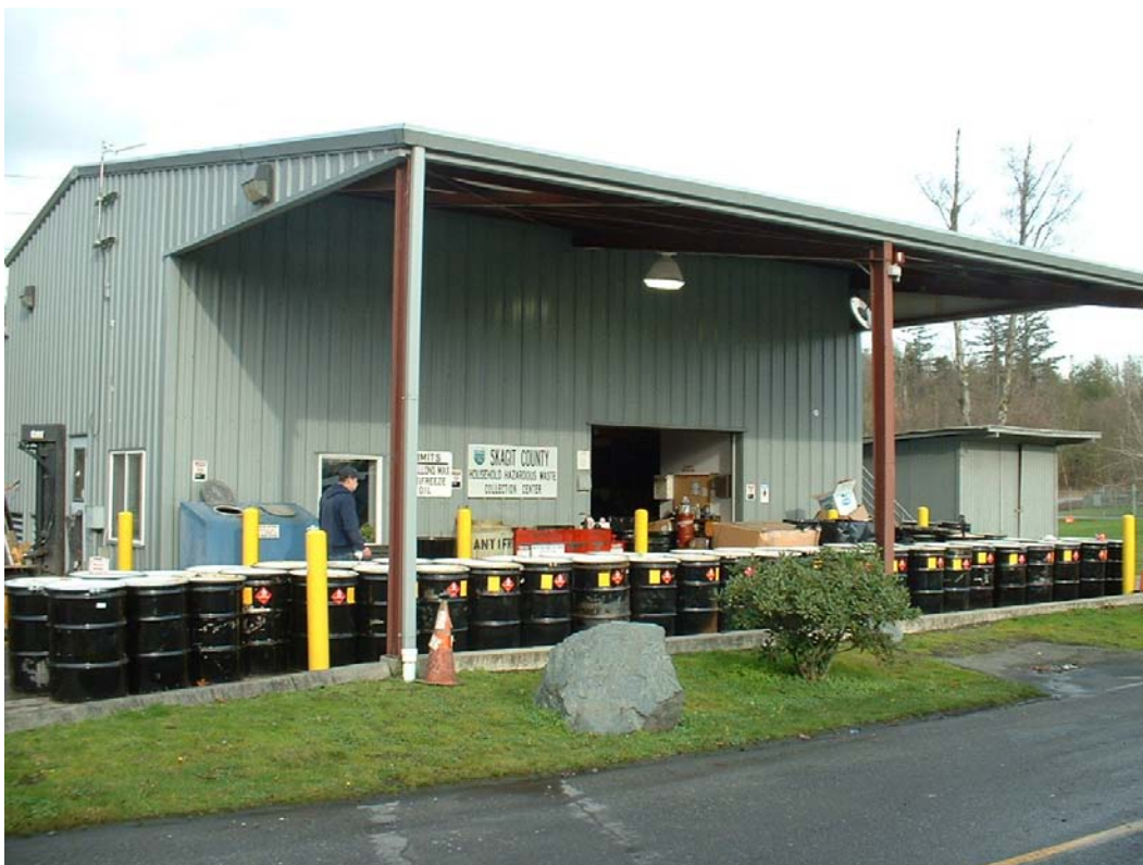
Figure 8 Moderate Risk Waste Facility
