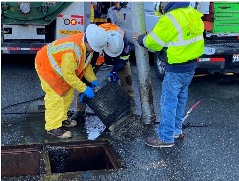
Figure 8-1. A crew replaces a stormwater filter in a catch basin at near Guemes Island Ferry Terminal.
