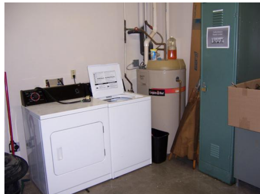
Lennox 'Complete Heat' hot water system is not working.
