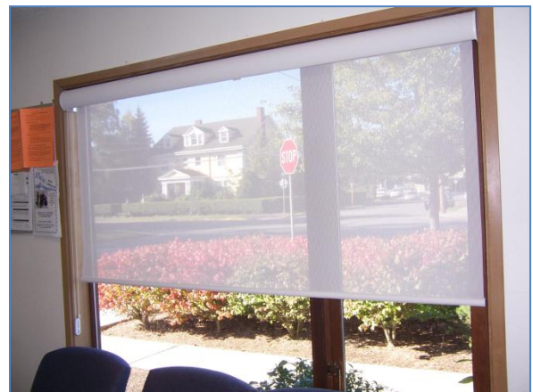
Nice solar-mesh shade on west-facing window in the reception area.
