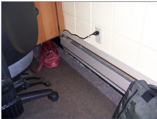
One of several baseboard heaters – some work and some don't.
