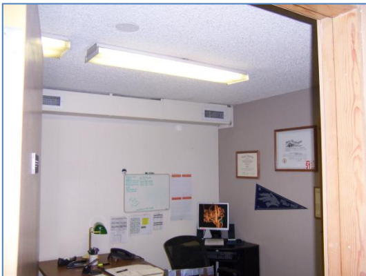
One of many unoccupied offices with lights left on
