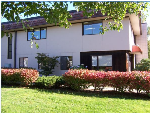
Upper, west-side windows have some roof-overhang protection from summer sun, but not the lower windows
