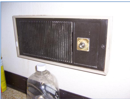
Electric wall heater with control knob on the unit.
