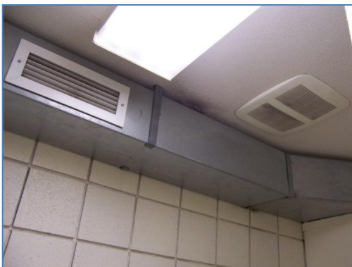
Restroom exhaust vent on the right is next to supply air coming into the space from the vent on the ducting.
